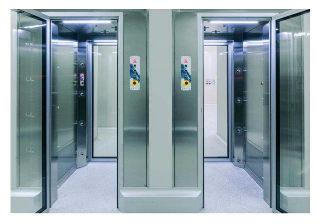
The air shower is employed to decontamine the clothing of the operator entering a controlled contamination room (cleanroom) or exiting from an area infected or contaminated with powders which must not propagate outside.
